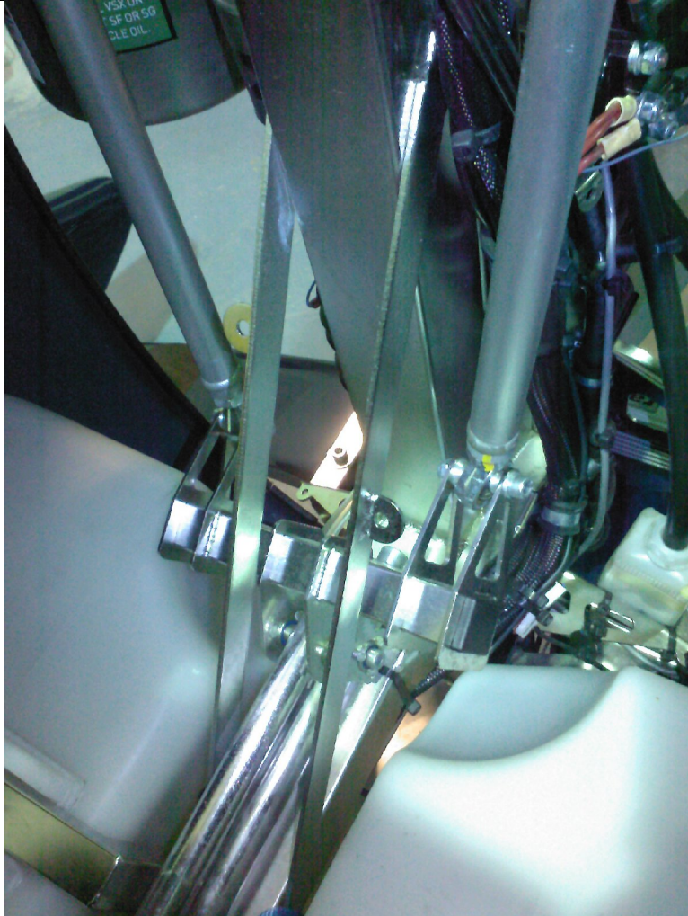
View of straps welded in place The straps are welded at 35 degrees to the mast.
