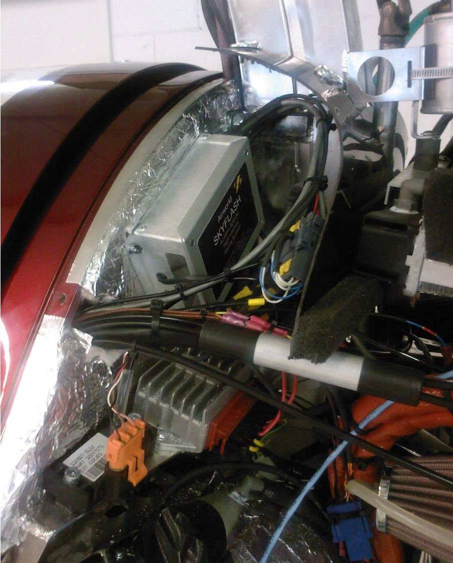
Skyflash control box location
