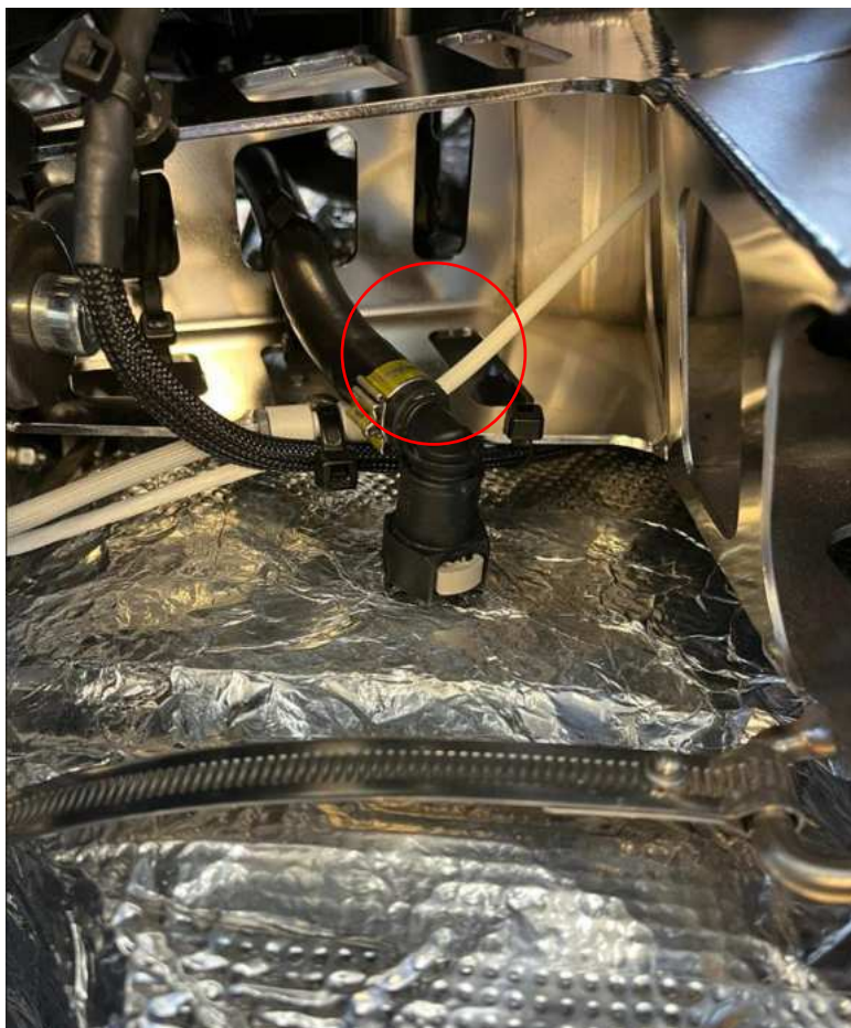
Figure 2 – Tank vent line needs to be disconnected
