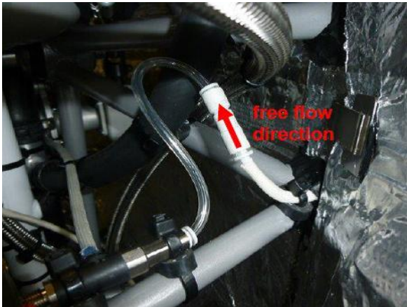
Fig. 3 - Connection of check valve to pressure reducer
