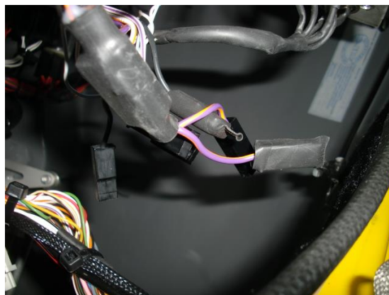
Fig. 4 - Isolation of cable end
