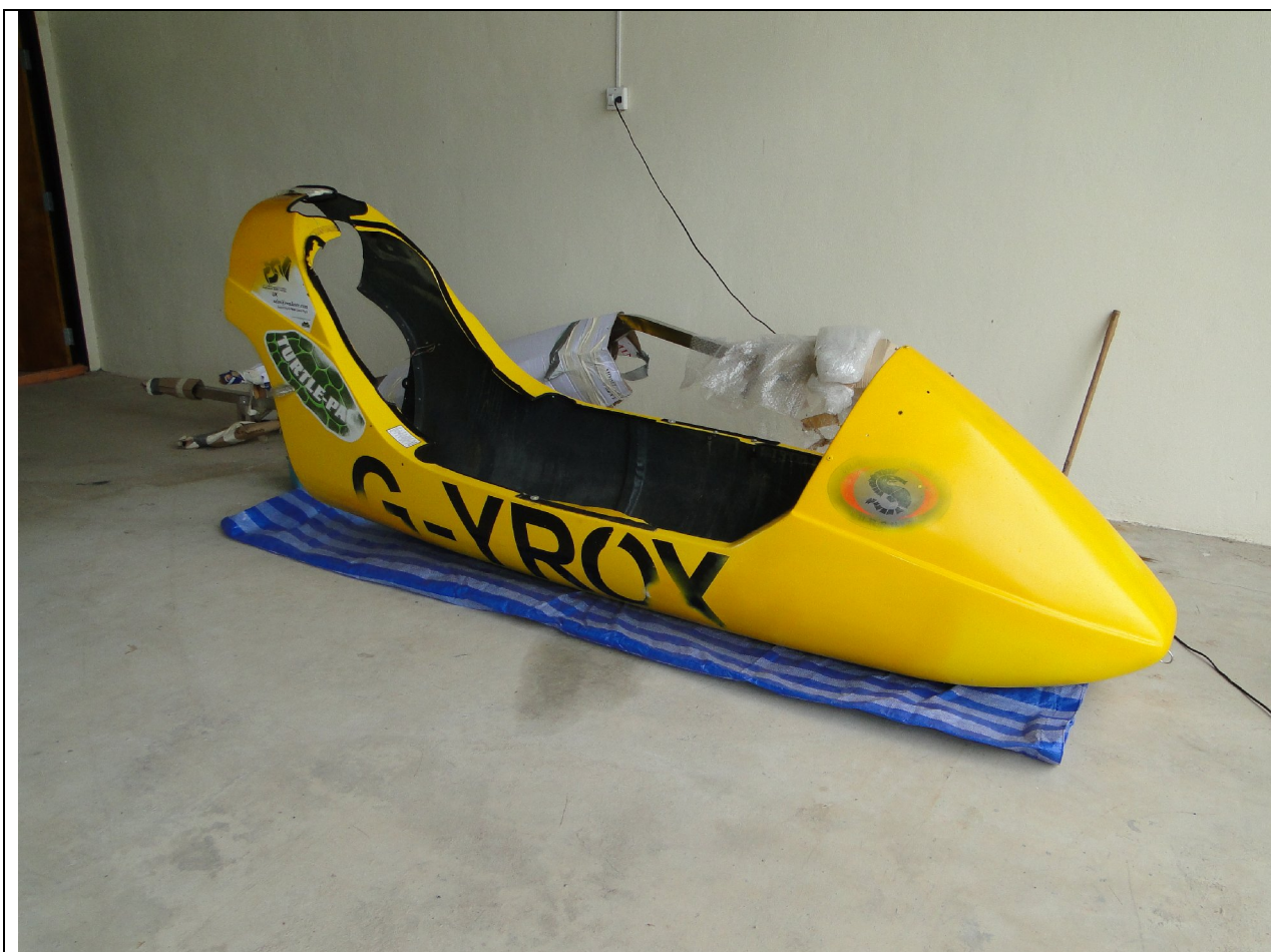
View of repaired enclosure. The paint is a rough match only, and has still to be cleaned off the registration letters
