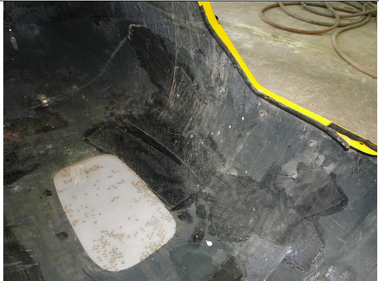
View of the repairs inside
