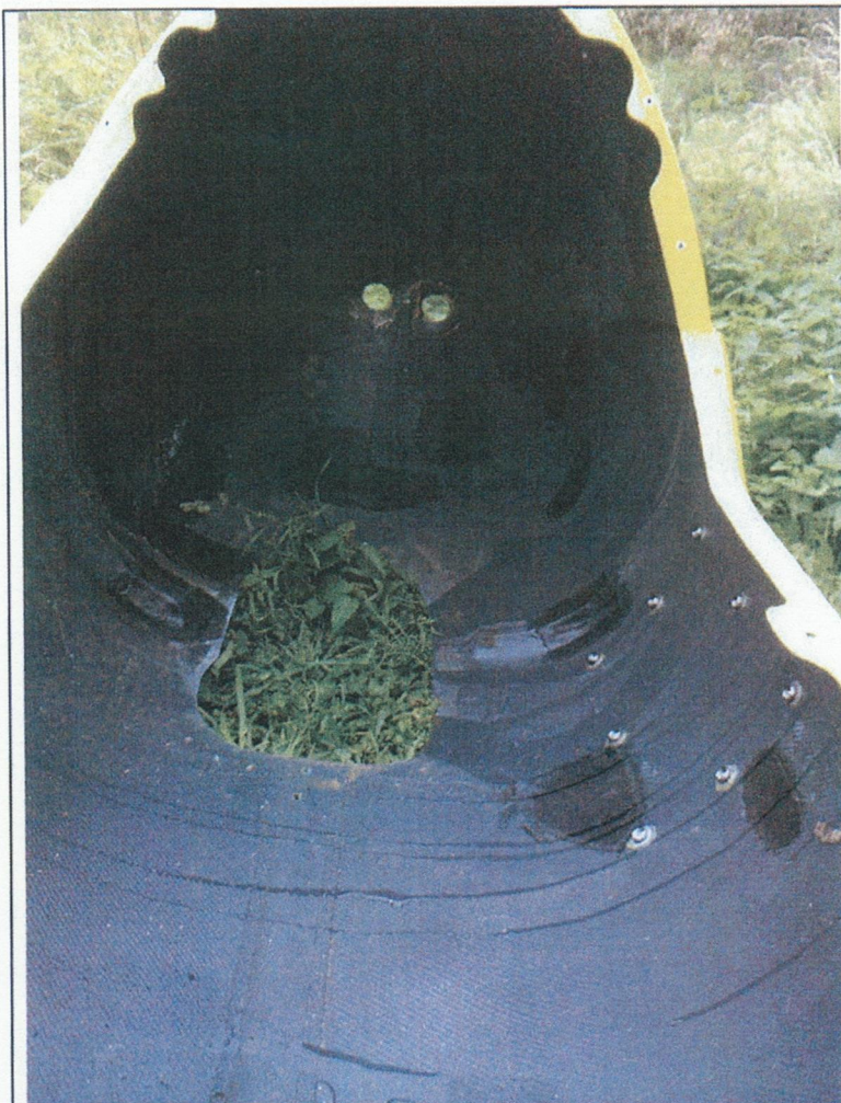
Inside of nose after repair
