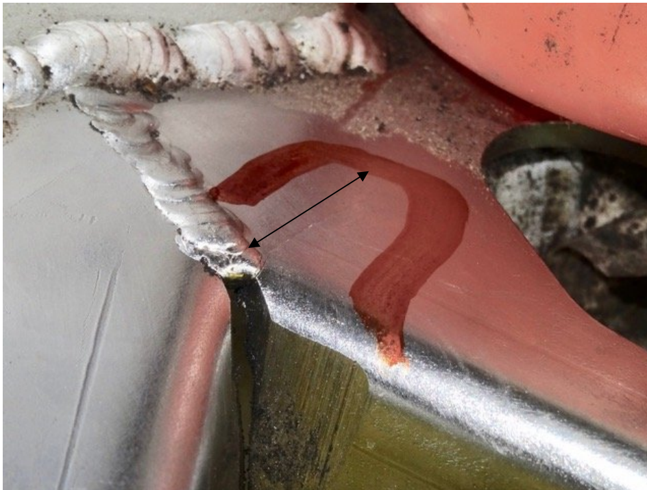
Short weld-run after preparation
